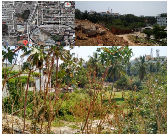
Fig. 3: Location map of Banashankari quarry site next to metro showing the current delapidated status
